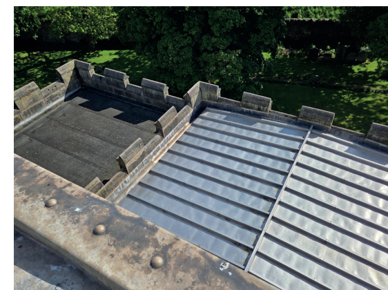
Left: Organ chamber roof Right: Sanctuary roof
