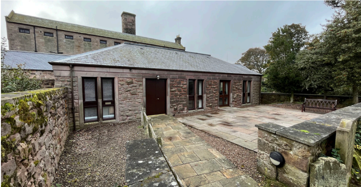
Exterior of the Parish Centre.
